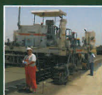
Airport paving: Airports around the world are gearing up facilities p31
