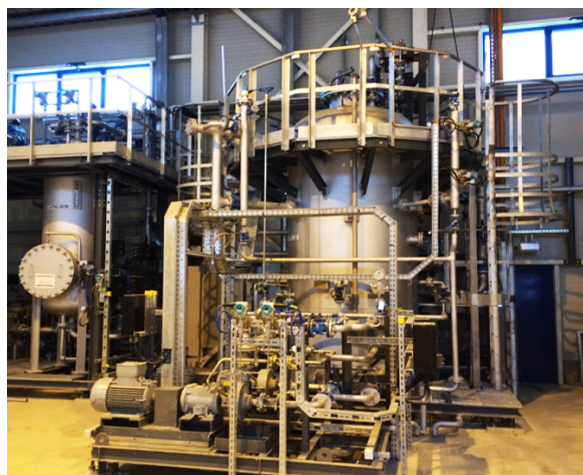
Supply and commissioning of a produced water treatment plant for subsequent injection into deposit with capacity of 41.6 m 3 /h (Tazlau / Romania, executed on behalf of Siemens)
