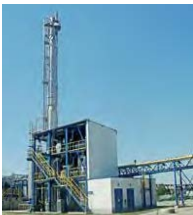
Formalin plant, Dynea Erkner GmbH, Germany, 2015
