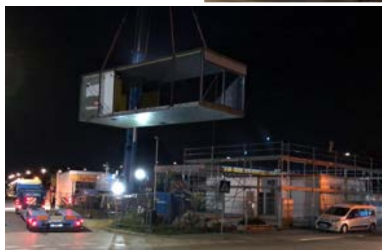
Overnight, a 350t crane lifts the modules (up to 4.90 x 13.10 x 3.85m and 31 tons) into position. Everything fits – in the morning, traffic flows again without disruption.
