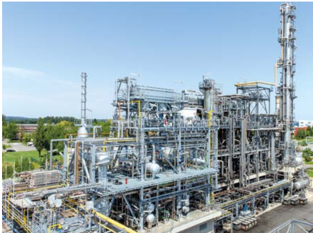
Existing used oil re-refining plant in the Zeitz Chemical Park – designed by EDL in 2010 and 2016
