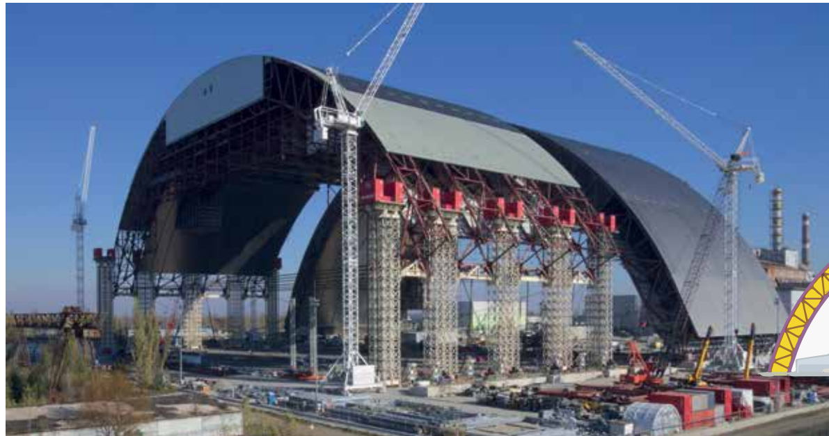
The work on the roofing over the damaged reactor in progress.
