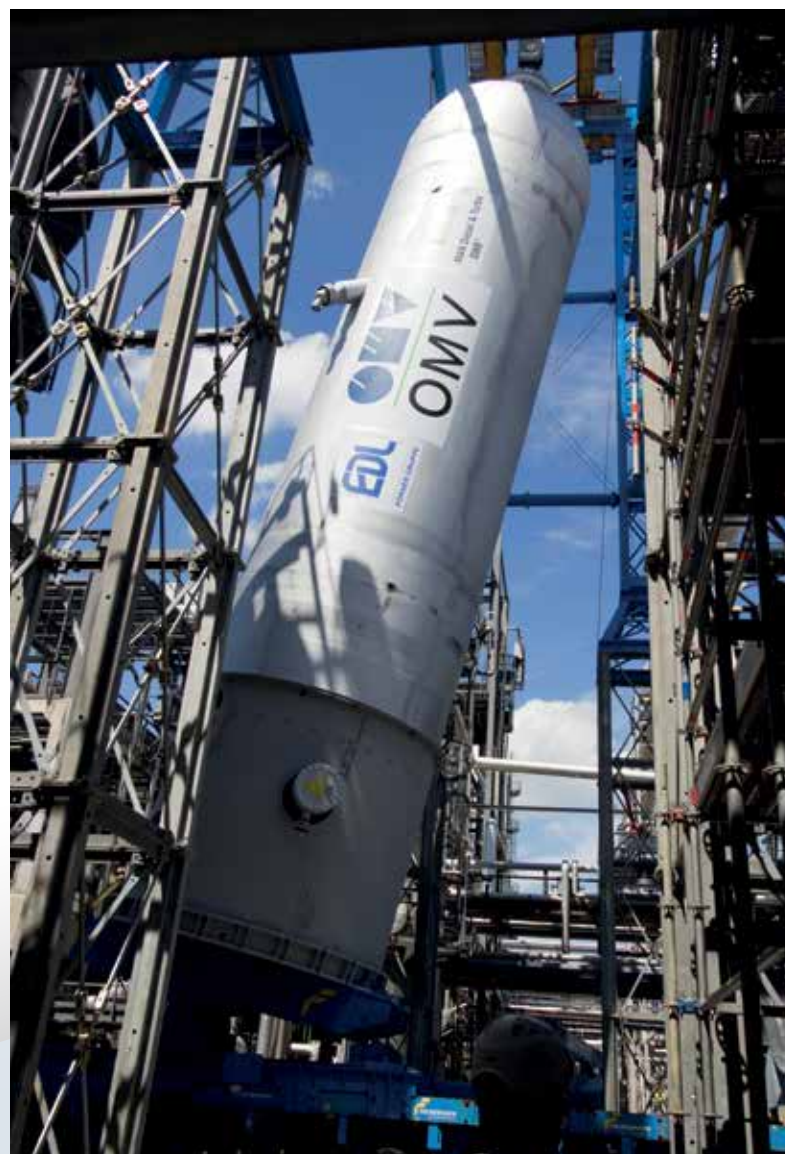
An uplifting experience: the new HDS3 reactor is erected and can be placed onto the foundation with no re-adjustment.
