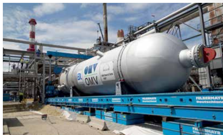
With a clearance of just 8 cm the reactor was shoved through under the pipe bridge on a special hydraulic unit.
