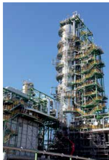
Mechanical completion of the vacuum column according schedule as part of the shutdown "kleiner 16", with 71 m in height and a total weight of 760 MT.
