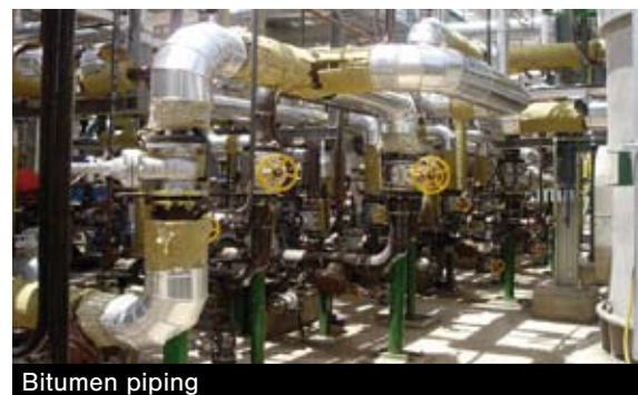
Bitumen piping
