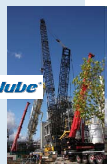
Placing of the colonne
