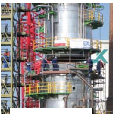
Assembly of column parts - everything goes acc. to schedule
