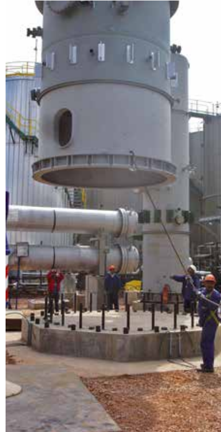
Biturox® plant SAMIR, Morocco, 2011
