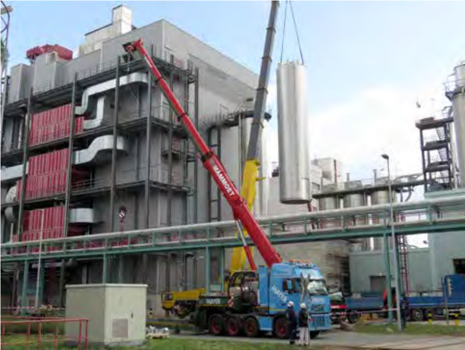
I.: An important milestone reached in September 2019: the silo for vehicle loading is installed without any complications. Based on a new loading technology transport vehicles are now filled. Because of the inclined position of the vehicle tank, it is filled to a significantly higher level than before, thus saving necessary truck transports while having the same production quantity. This saves approx. 150 trucks per year! A great contribution to reduce costs and protect the environment!
