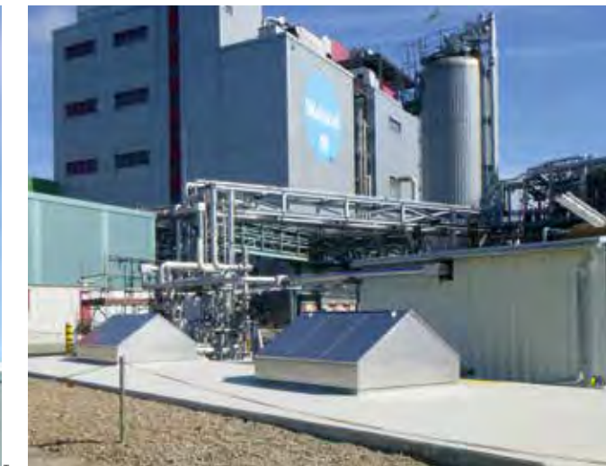
a.: The ethylene oxide tank is buried and safely covered. The last step in the overall project is completed! A reduced number of ethylene oxide loading operations from tank wagons into the new underground ethylene oxide tank leads to a lower risk for overall rail traffic, since fewer tank wagons with dangerous goods are on the way.
