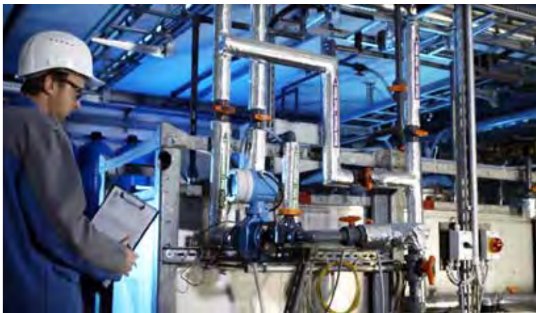
Demonstration plant in Freiberg / Germany provides evidence of purity.
