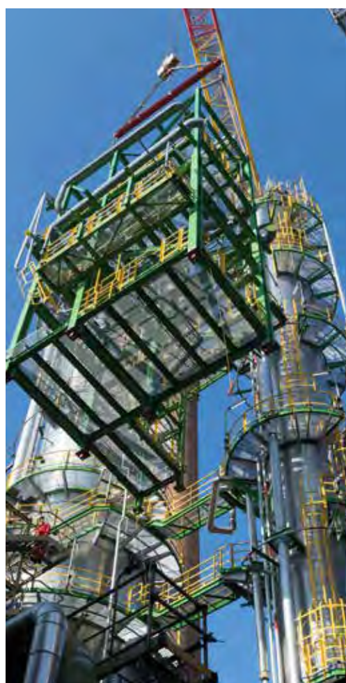
New column K3 of the crude oil plant is being lifted
